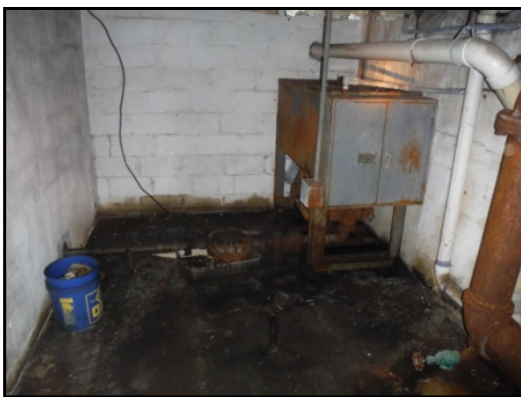
35 : Freight elevator equipment room (staining)
