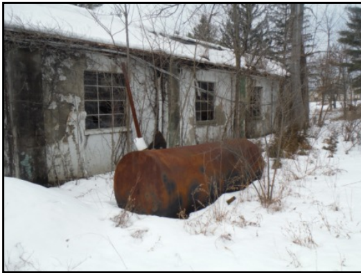
37 : Excavated UST (Maintenance Warehouse)
