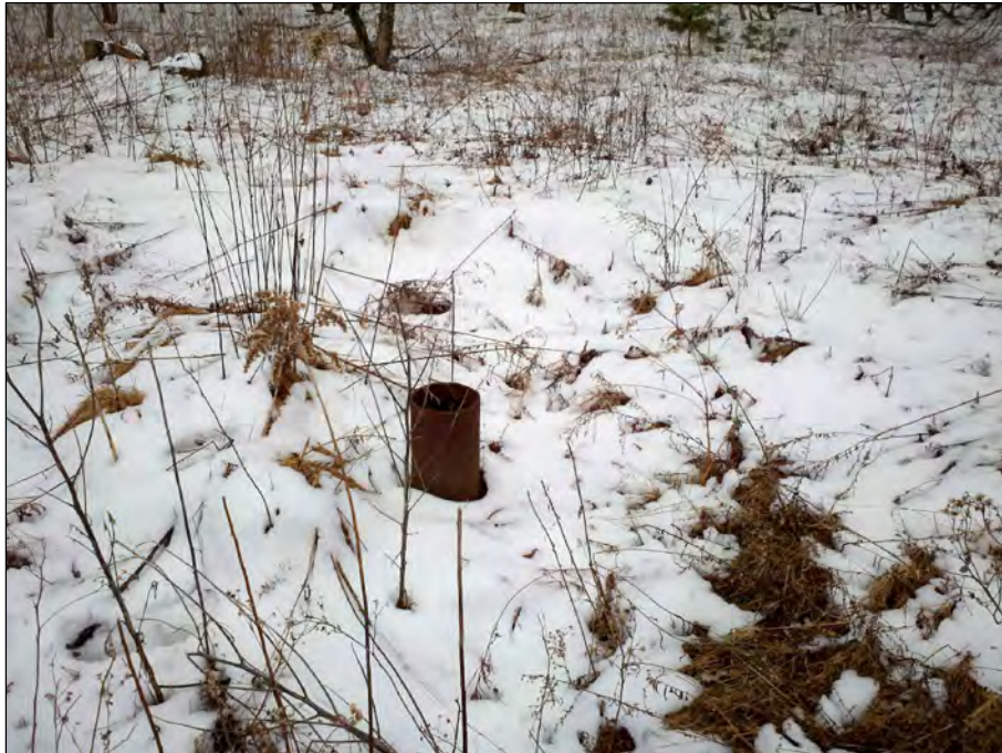
1. EXISTING WELL 20 ON EAST SIDE OF JOYLAND ROAD, NO WELL PUMP AND NO WELL CAP.
